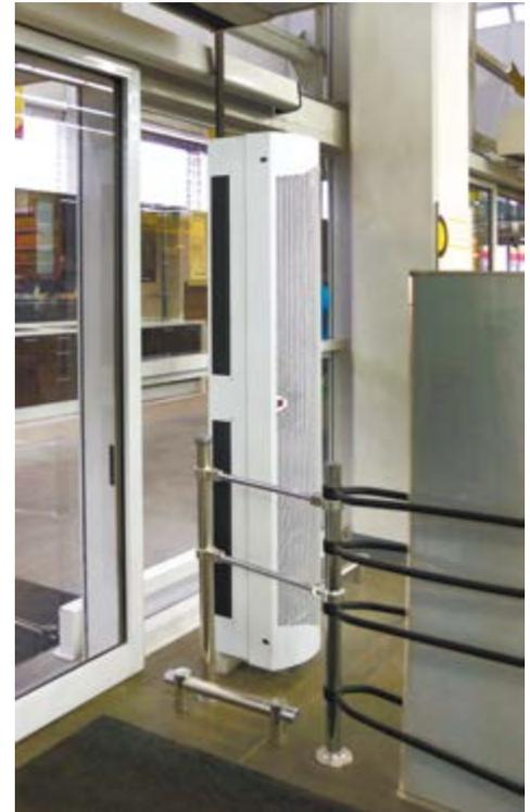
Series 400 – Higher output units for high pedestrian traffic areas, larger volume buildings i.e. malls, recreational facilities, smaller warehouse bay doors. Available heated (electric or water) or unheated. Versatile in many different commercial or industrial applications. Control panel included with every air curtain. Complete with - 3 speed control, Thermostat and 2 heat settings.
